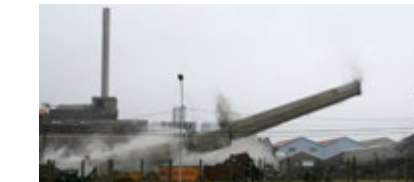
Providing for the demolition of a concrete chimney, Corbehem
