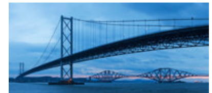
Involved in the new Forth Replacement Crossing, Scotland
