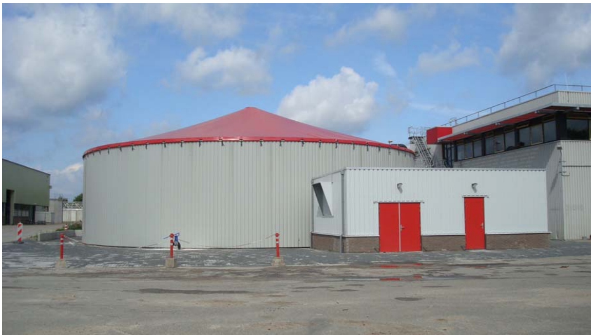
Figure 3 DEMON system at Apeldoorn WWTP
